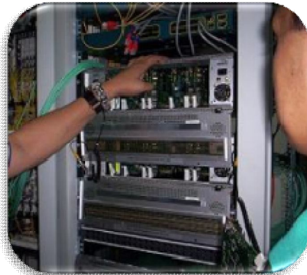
Installation of CWDM Fiber Module at Astro Measat Cyberjaya
